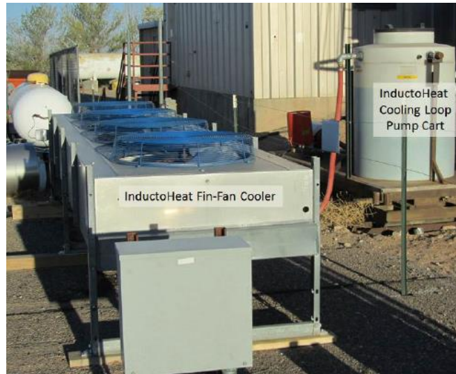
Figure 2.5. a. Electronics enclosure with InductoHeat controller, pyrometer, and heat exchanger, and b. connected cooling loop and cooler [36].
